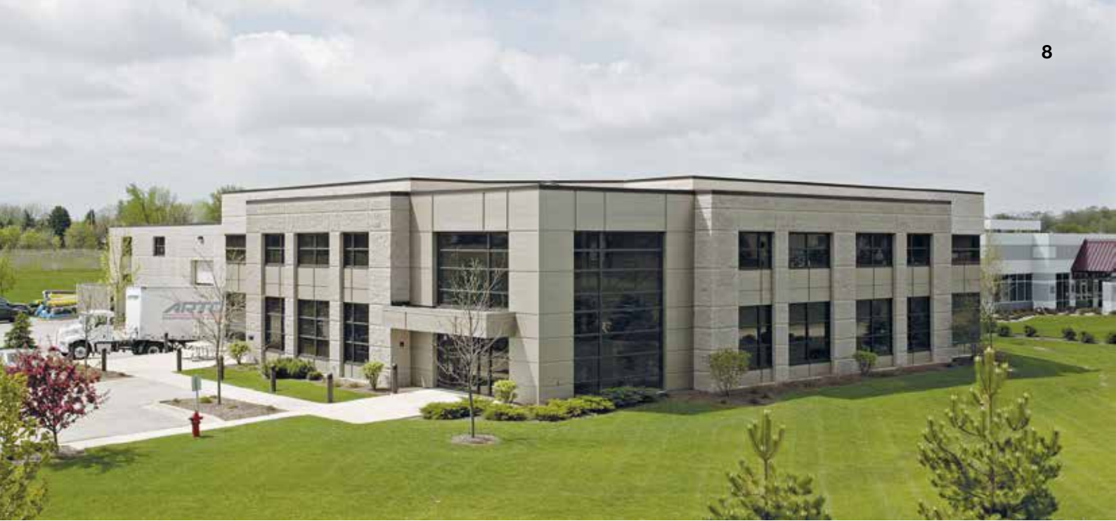
Artos Engineering in Brookfield, Wisconsin, USA
